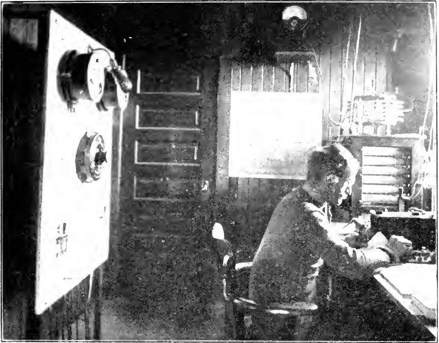
THE INTERIOR OF A HIGH POWER STATION
